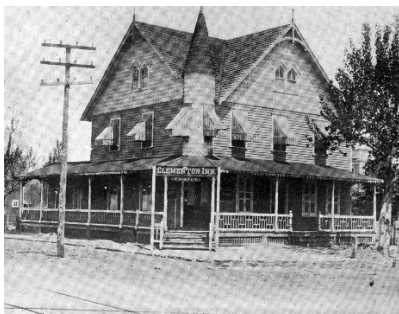
Fred Ribaut's original Clementon Inn, destroyed by fire in 1911. A plaque reading "F. Ribaut" hangs beneath the "Clementon Inn" sign.
