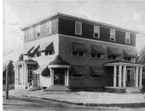
The rebuilt Clementon Inn in an undated photo.
